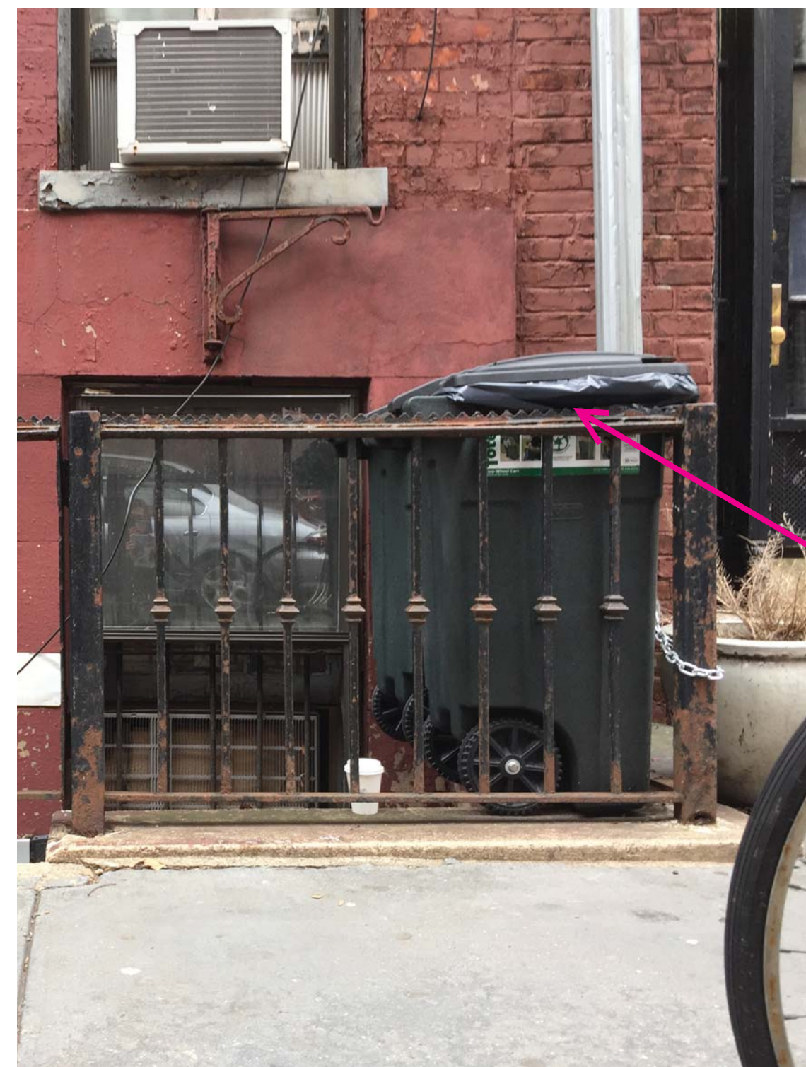
RAILING AT 182 WAVERLY PLACE (SQUARE COLLARS & RODS)
